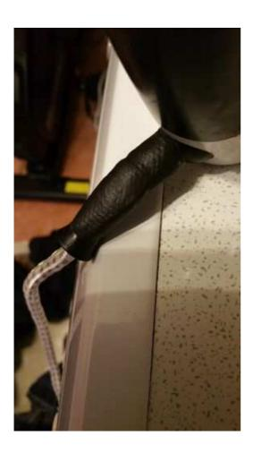
In the picture above, showing the repair to an iron, the black patterned 'sausage' has been moulded over the original cable support mesh, which broke. I've now heard of a guy who used it to repair a battery connection pillar. He broke it trying to undo a corroded bolt but moulded Sugru over the area that should be attached to the battery. Got him out of trouble.
